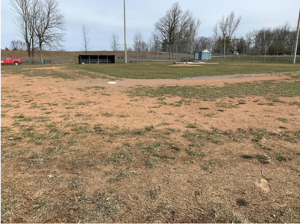
The warning track is overgrown with grass. Infield skin installation and grading is needed.
