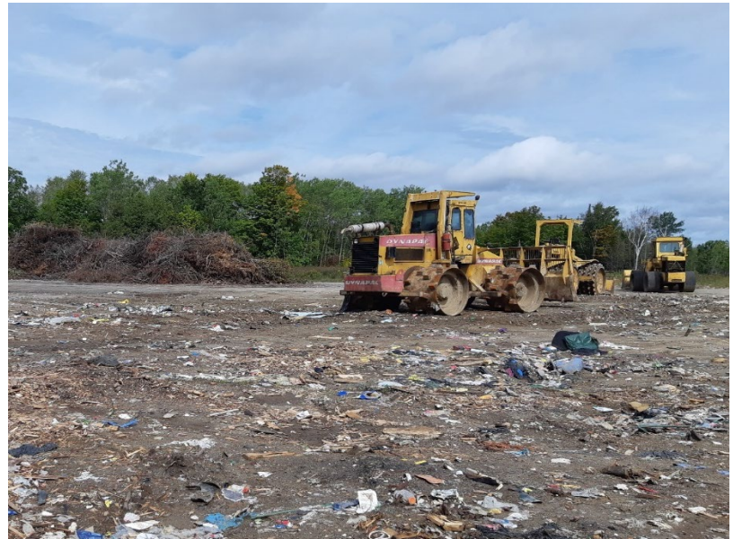
Figure 4 Garbage Compaction Equipment – McDonald's Corners WDS
